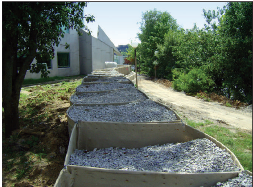
Figure 3-6. Gravel-filled containers formed a barrier to protect University of Iowa facilities during a flood event (2008).
