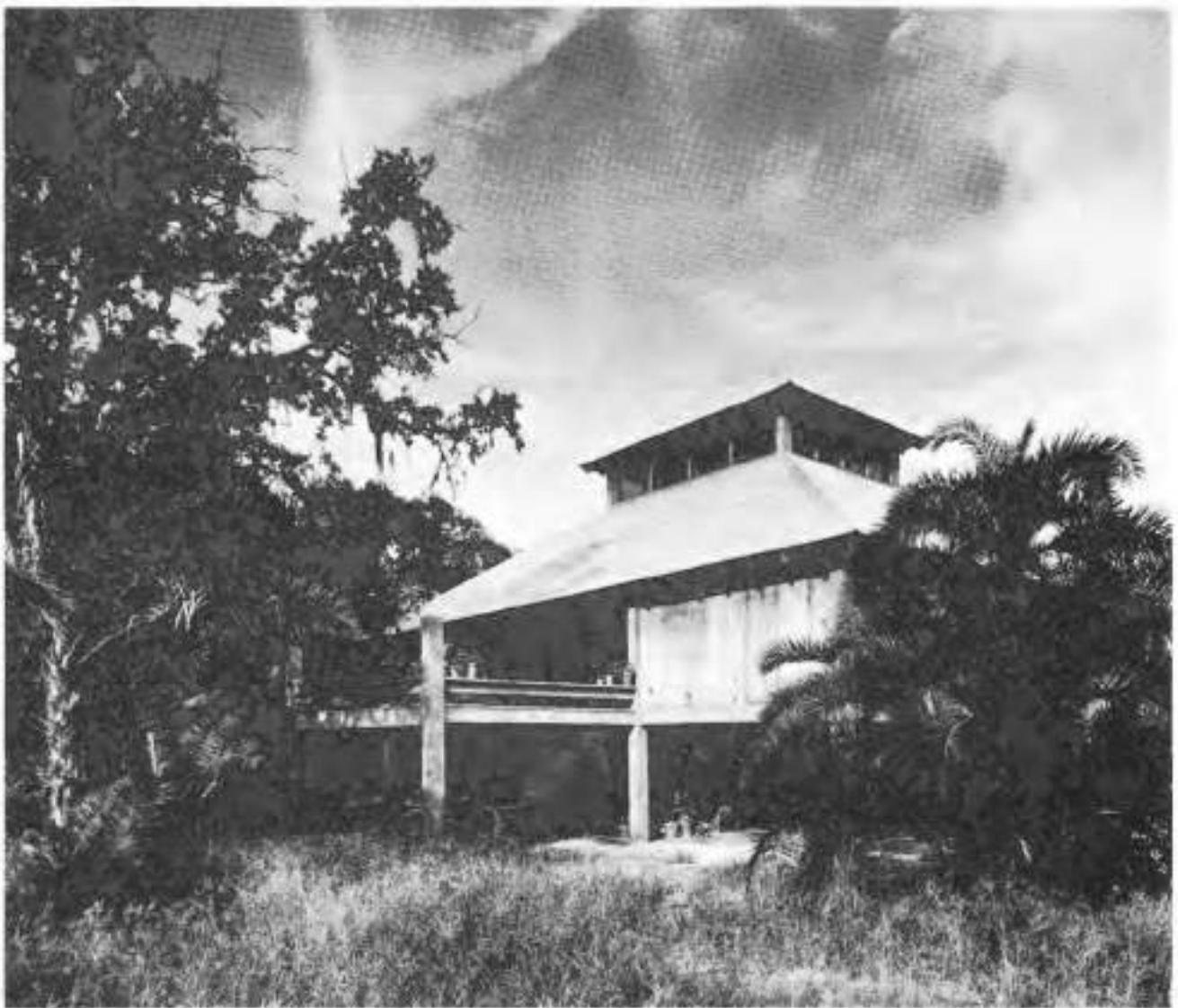
Figure 3.31. This is a good example of how a simple structural grid infrastructure can be used as a basis for a relatively modest, well-designed and visually appealing residence. The plan is simple, developed around the columns, but provides a very livable, interesting and functional space. The cantilevered balconies also add interest as well as defined exterior areas. The roof shape contributes to a spacious interior that makes the house feel larger than it really is, allows in natural light through the transom windows, and through its form adds much to the overall aesthetic appeal of the design (see also Figures 3.40 through 3.45).
