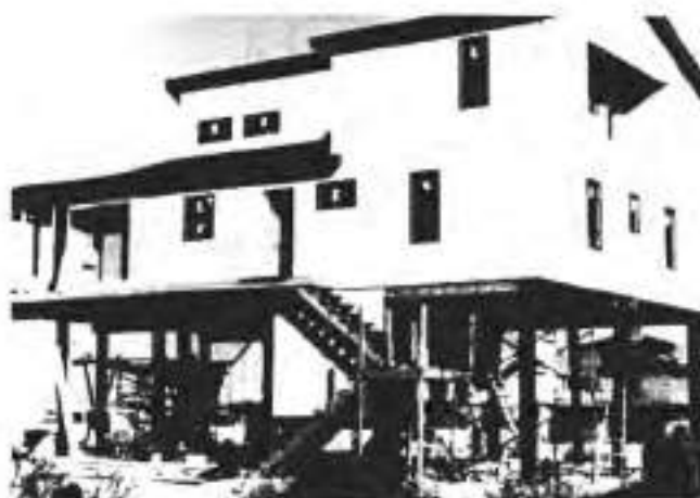
Figure 4.14. Pile Foundations
