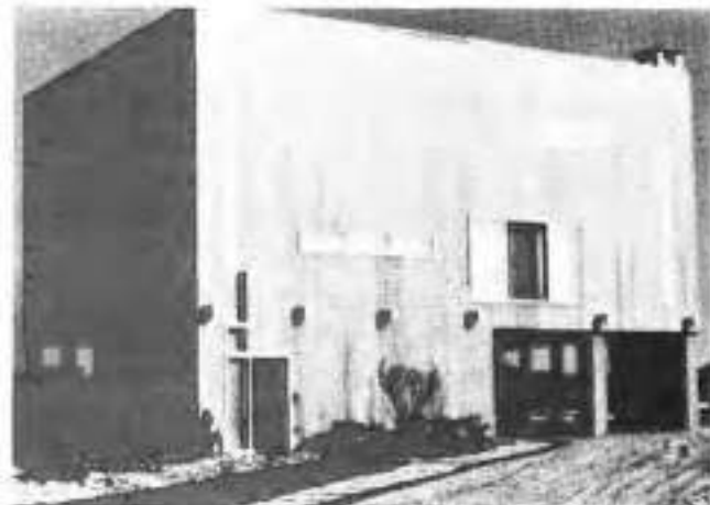
Figure 3.26. This is an example of integrating the site, the building, and the foundation so they relate well to each other. This foundation appears to be part of the building rather than stilts holding it up. It shows how a modest, simply designed building can also be very aesthetically appealing through the use of natural materials and interesting treatment of fenestration and lighting fixtures. Simple but well-thought-out landscaping ties the building effectively to the site.
