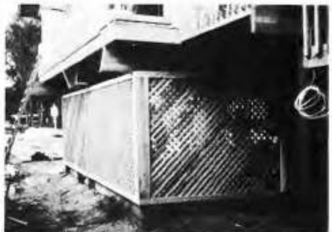
Figure 4.54. Breakaway Walls
