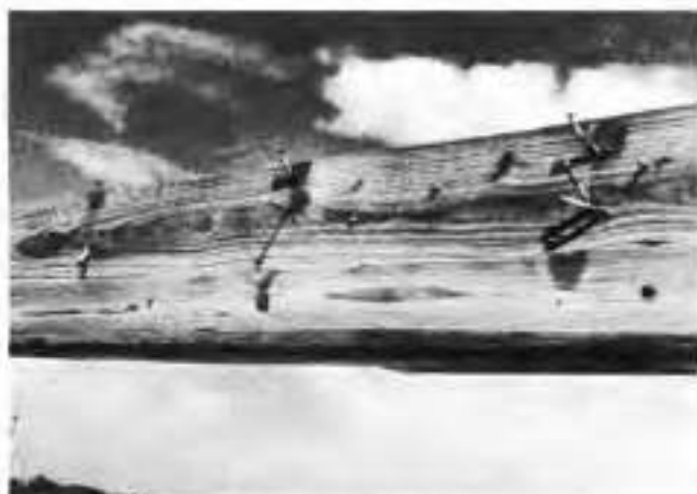
Figure 4.26. Toe Nailing Provides Limited Pull-Out Resistance
