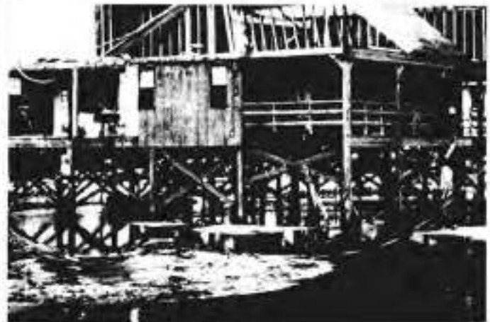
Figure 4.23. Diagonal Bracing
