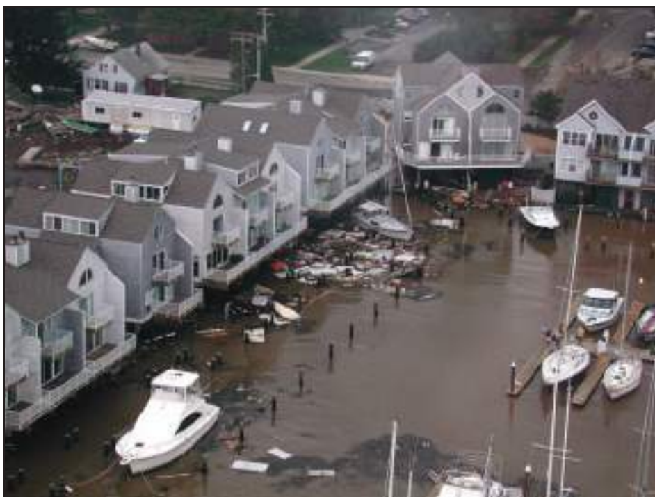
Figure 4-21. Condominiums built along the shoreline at the mouth of the Susquehanna River on the Chesapeake Bay were subjected to flood-borne debris after Hurricane Isabel (Havre de Grace, MD, 2003)
