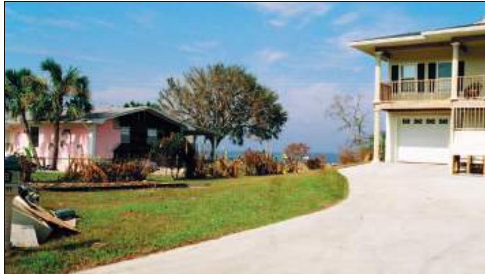
Figure 2-15. The pre-FIRM house (left) experienced damage due to surge and waves while the newer, elevated, post-FIRM house (right) experienced minimal damage, Hurricane Ivan (Santa Marina, Pensacola, FL, 2005)
