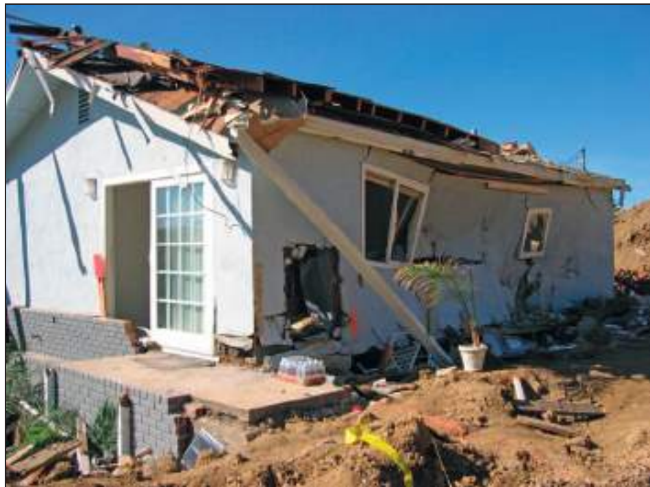
Figure 2-8. This building experienced structural damage due to a landslide in La Conchita, CA, after a January 2005 storm event
