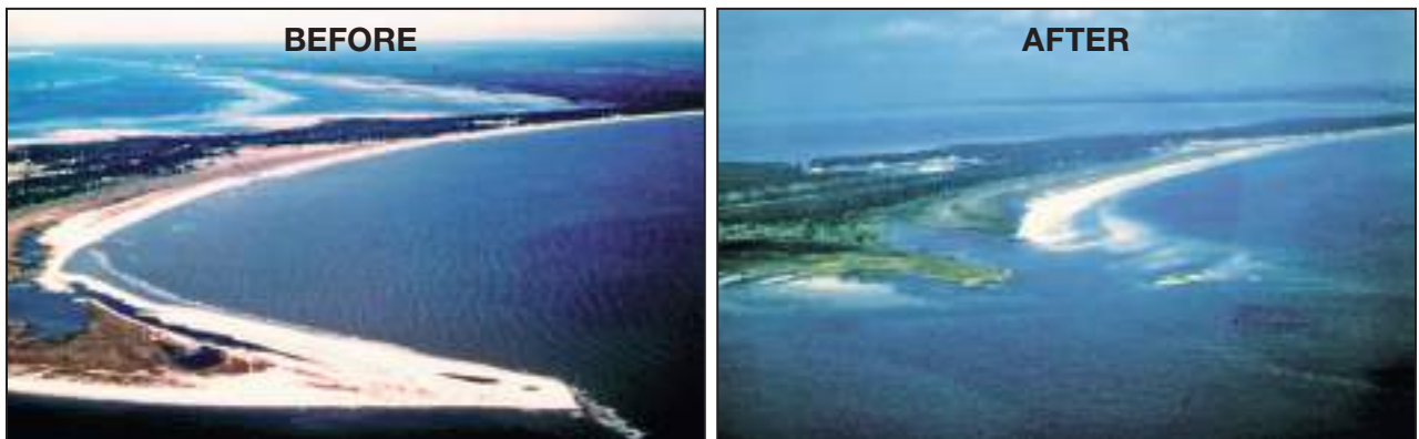
Figure 3-40. Cape San Blas, Gulf County, FL, in November 1984, before and after storm-induced erosion
