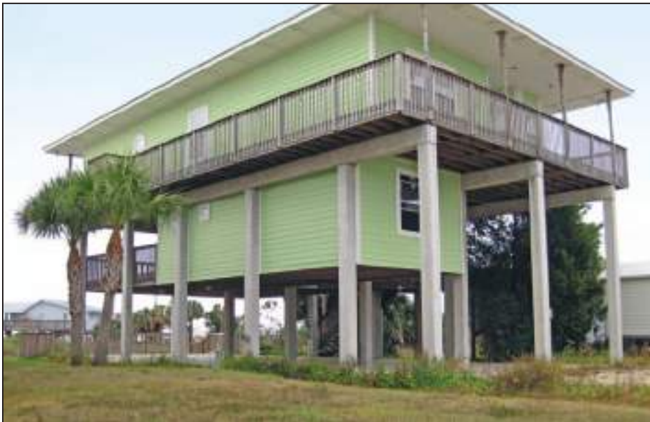
Figure 2-23. Above-grade enclosure (Perry, FL)
