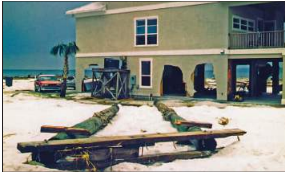
Figure 3-28. Pier pilings were carried over 2 miles by storm surge and waves before they came to rest against this elevated house in Pensacola Beach, FL (Hurricane Opal, 1995)
