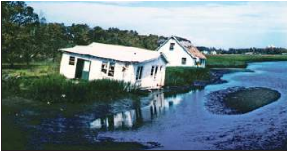
Figure 3-18. Intact houses floated off their foundations and carried inland during Hurricane Hugo in 1989 (Garden City, SC)
