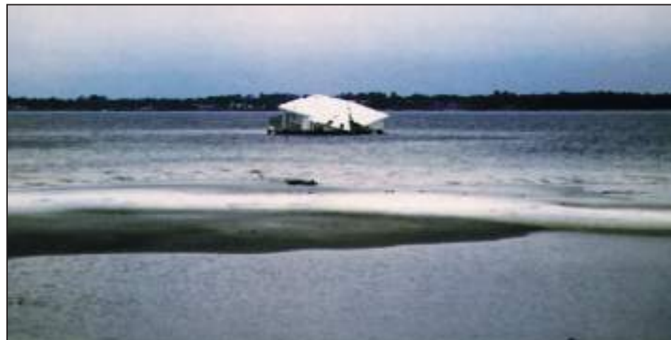
Figure 3-22. This house, located in an area of channeled flow near that shown in Figure 3-20, was undermined, washed into the bay behind the barrier island, and became a threat to navigation
