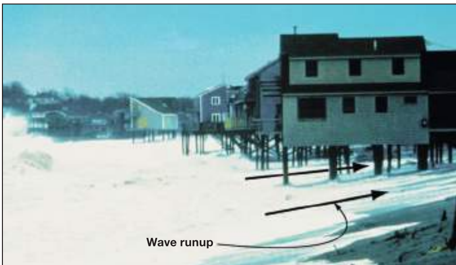
Figure 3-24. Wave runup beneath elevated buildings at Scituate, MA, during the December 1992 nor'easter storm
