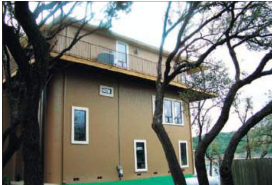
Figure 2-24. Two-story enclosure SOURCE: FEMA P-499 2010
