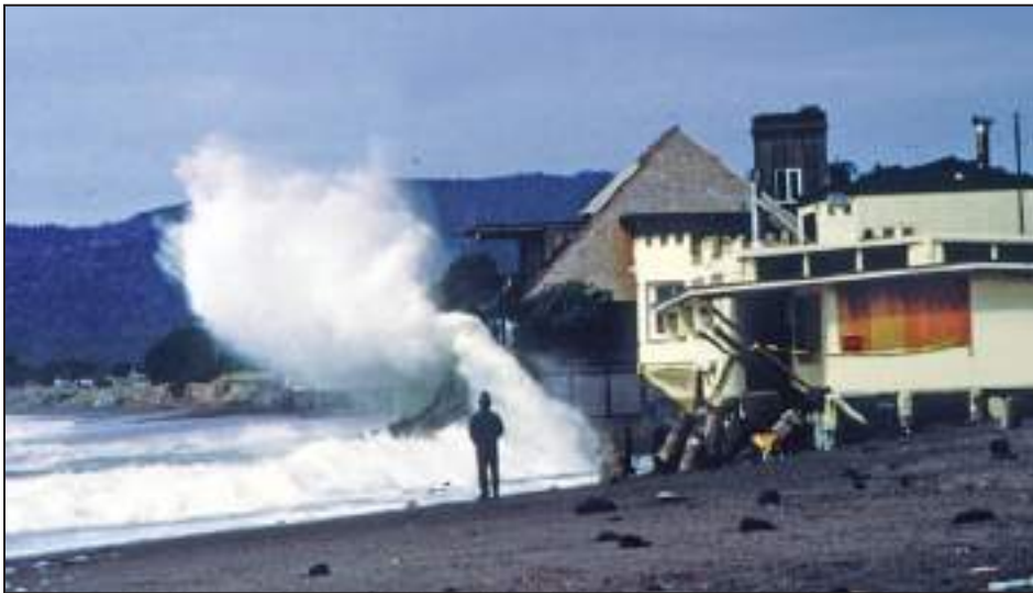
Figure 3-23. Storm waves breaking against a seawall in front of a coastal residence at Stinson Beach, CA
