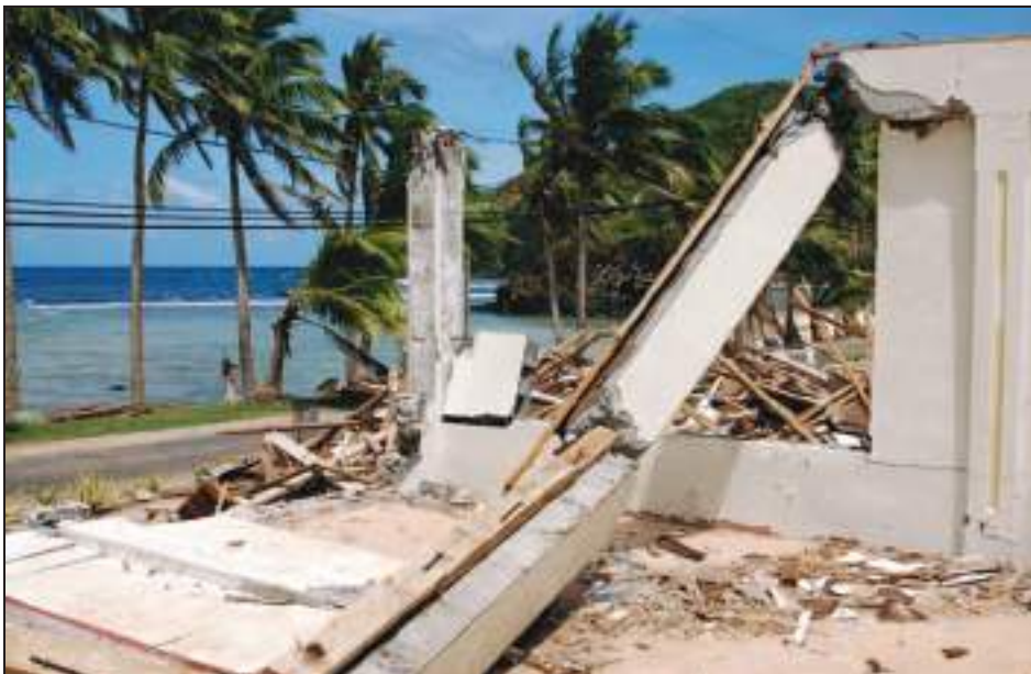
Figure 3-12. Damage from the 2009 tsunami (Amanave, American Samoa)
