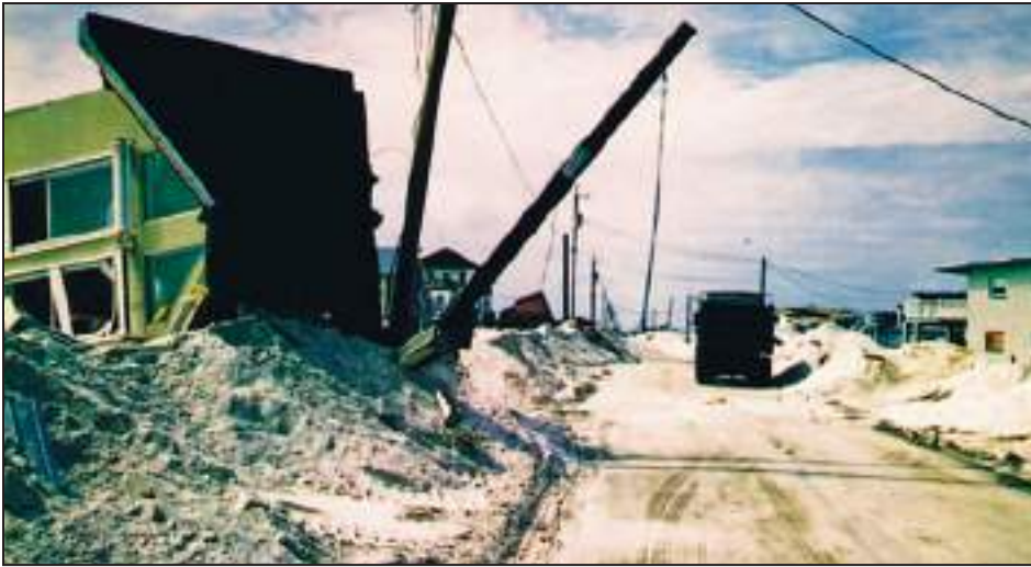
Figure 3-50. Overwash from Hurricane Opal (1995) at Pensacola Beach, FL, moved sand landward from the beach and buried the road, adjacent lots, and some at-grade buildings to a depth of 3 to 4 feet
