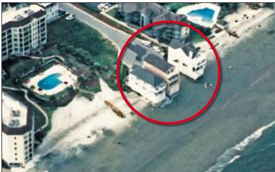
Figure 4-20. Three 2-year-old South Carolina houses left standing on the beach as a result of rapid erosion associated with a nearby tidal inlet (July 1997)
